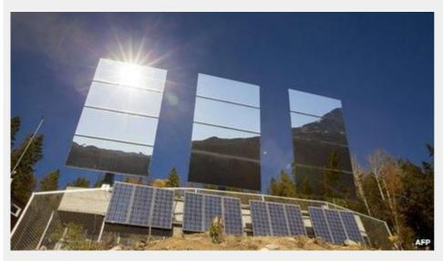
The three mirrors are controlled by computer and follow the path of the sun.
